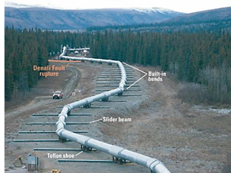
Figure 1. Oil pipe failure due to south central Alaska earthquake [3].
