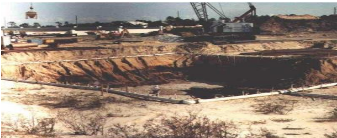
Figure 1. Construction well points system dewatering.
