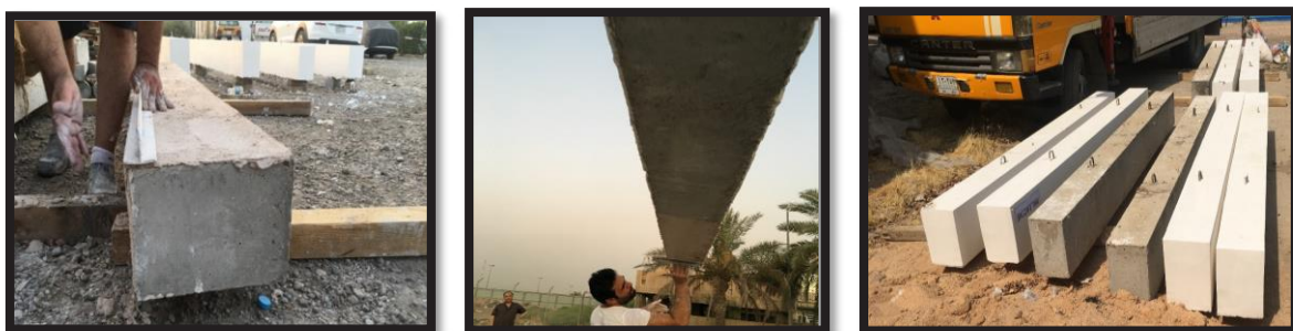
Figure 4. The specimens are covering with gypsum and plaster.
