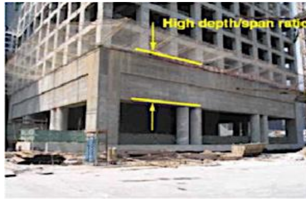
Figure 1. Photo picture of RCCDB [5].
