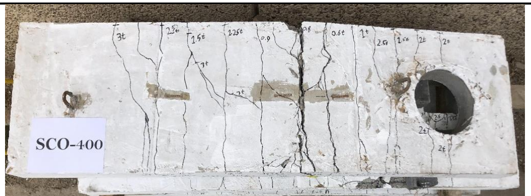
Figure 5. Cracks of SCO-400 slab.
