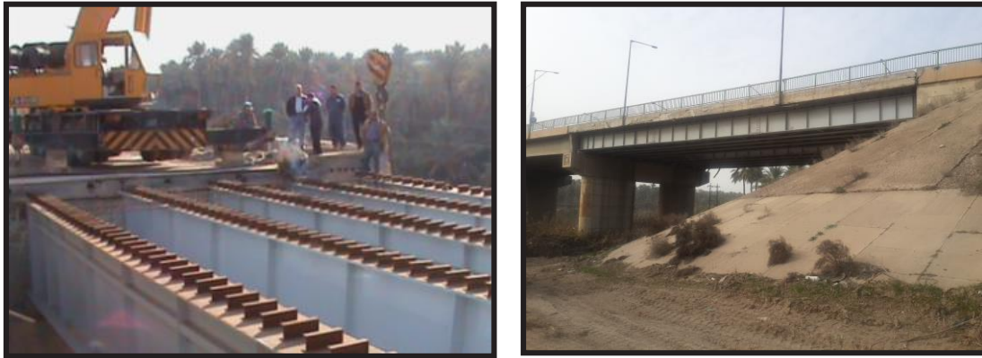
Figure 12. Al SABIYA Bridge.
