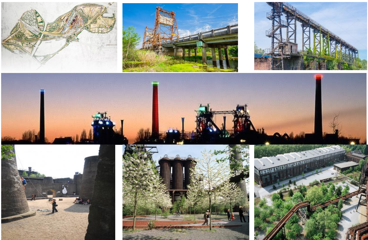
Figure 6. Showing the giant mechanisms and facilities at the site before the project. [19,20].
