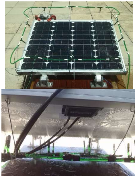
Fig. 14. The water spraying cooling of PV module [47]
