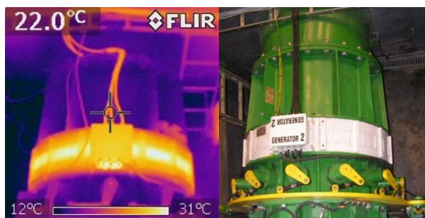
Fig. 6 Temperature distribution of the stator of the integrated hydro unit (the stator temperature at rated load did not exceed 36 ° C)
