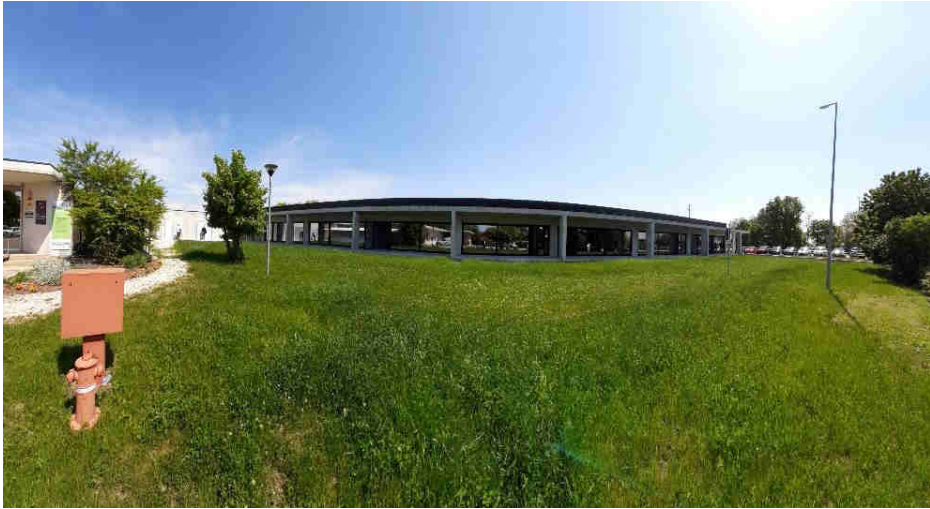
Fig. 2. Image of the new extension part of the school
