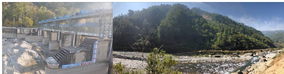
Fig. 1. Left: Gola Barrage at Kathgodam – Right: Jamrani dam site – Left abutment view from the right bank (source: ADB).
