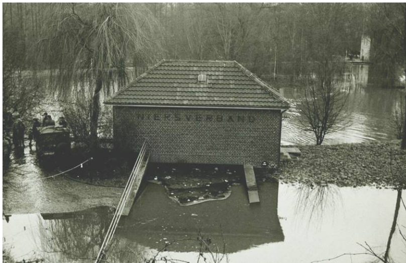
Fig. 1. Picture of outlet structure during the flood 1963 – the flood water level reached the dam crest.
