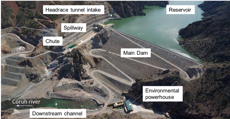
Fig. 2. Downstream view of the main dam with environmental powerhouse on the right side of the picture (Source: EnerjiSA).
