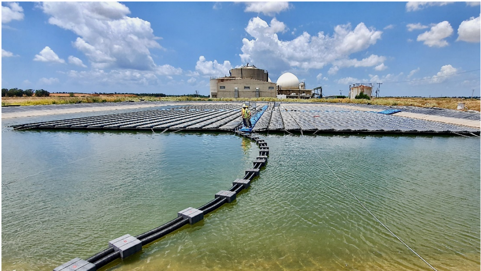
Fig. 4. Hefer: FPV system under final inspection.
