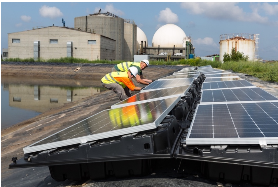
Fig. 2. Preparing to lower the 5° tilt FPV panels and floaters into Hefer reservoir.
