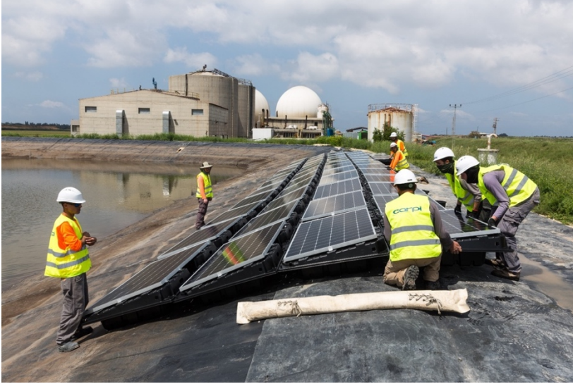
Fig. 3. Lowering the FPV panels into the reservoir.
