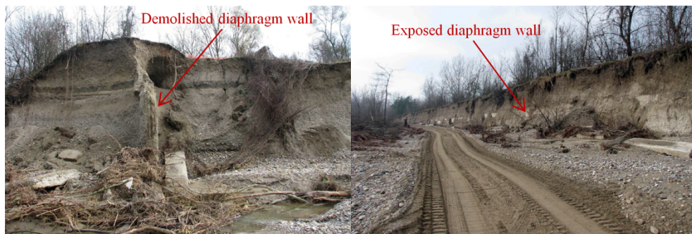
Fig. 15. Demolished and exposed diaphragm walls (Photos: A. Geršak).
