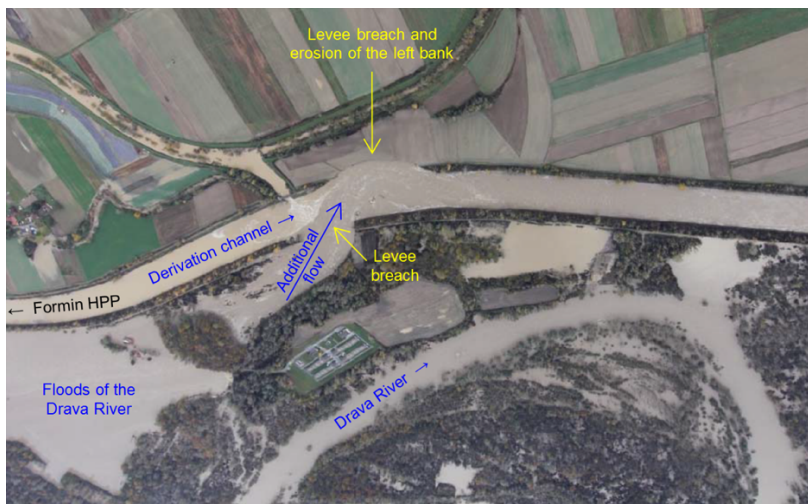
Fig. 12. The area with the greatest damage - during flooding (Photo: Mensuras photo archive).
