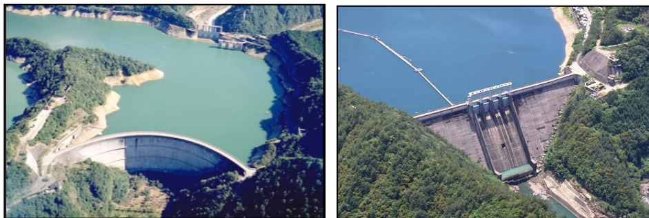
Fig. 2. Ikehara Dam(left) and Kazeya Dam(right).
