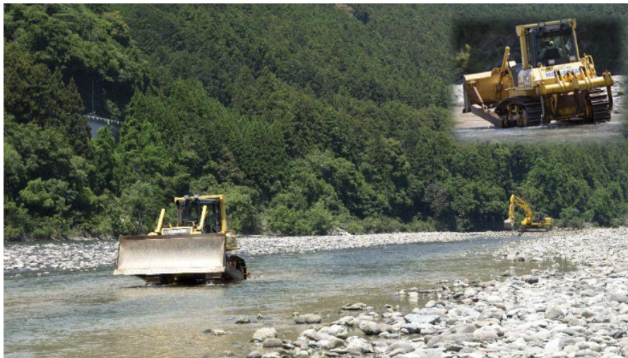
Fig. 6. State of river-bed tilling using a bulldozer's ripper on May 24, 2019.
