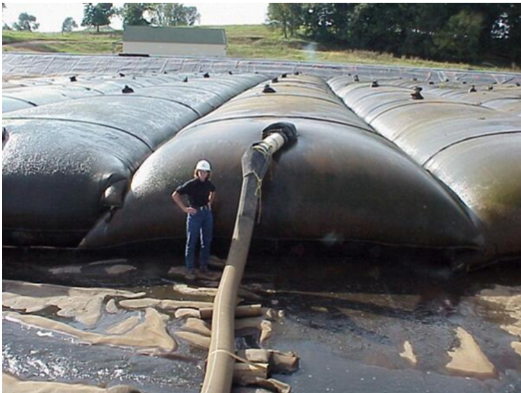
Fig. 7. Dewatering sediment bags.
