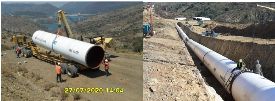
Fig. 6. Pipes of diameter 1800 mm to 2500 mm.
