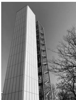
Fig. 4. High-rise demonstrator and access tower
