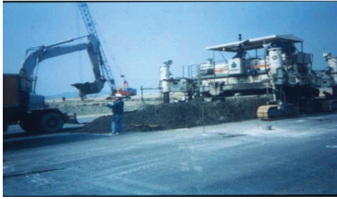
(a) construction photo
