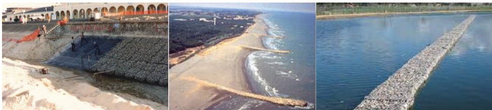
Fig. 5. Examples of revetments, groins and breakwaters built with steel mesh geocontainers
