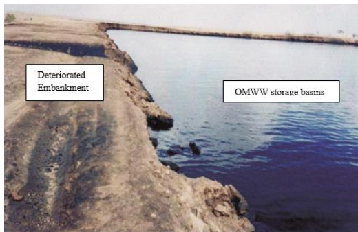
Fig.4. Deteriorated embankment
