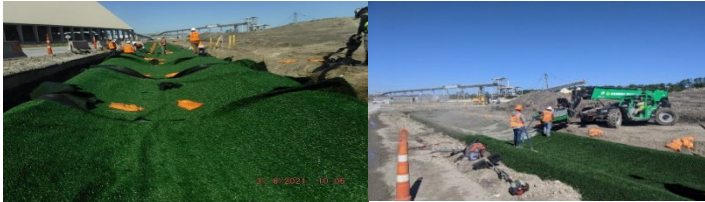
Fig. 7. Installation of synthetic turf and cementitious infill in the West Ditch.
