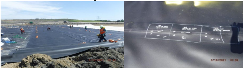
Fig. 6. Installation of the 1.5-mm thick geomembrane in the Sedimentation Pond.
