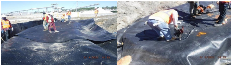
Fig. 5. Installation of the 1.25-mm thick geomembrane in the West Ditch.
