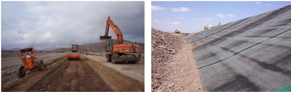
Fig. 4. Installation of BGM in Saday dike (Source: Axter)
