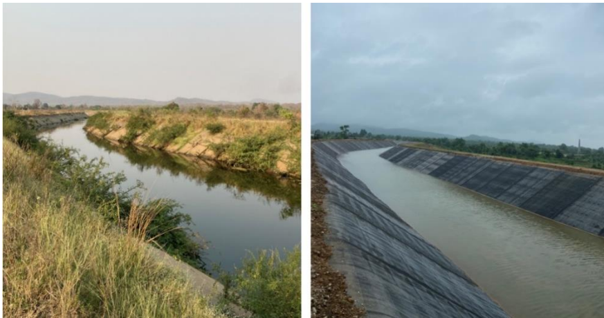
Fig. 9. Canal before and after renovation work - Pench Left Canal, India (Source: Axter)
