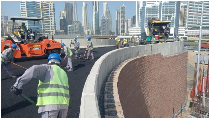
Fig. 8. Completed modular block wall in Business Bay, Dubai, U.A.E.
