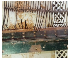
Fig. 8. GG1 failure when clamp is lined with sandpaper.
