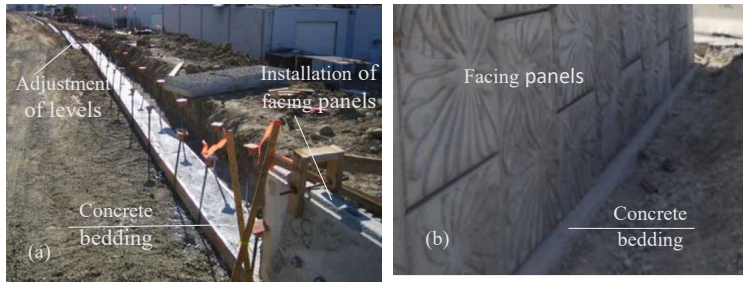
Fig. 1. (a) Concrete bedding preparation. (b) Facing panels installed on concrete bedding.
