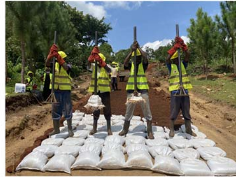
Fig. 2. Construction with Do-nou method in Uganda.
