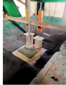
Fig. 5. Loading Configuration Installation
