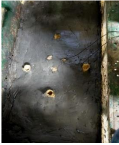
Fig. 4. After Columns Installation
