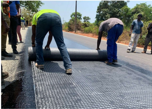
Fig. 6: PGL-G 100/100 installed over tack coat
