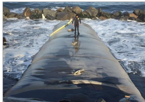
Figure 2: left: Initial filling of a tube; right: tube filling with diver support
