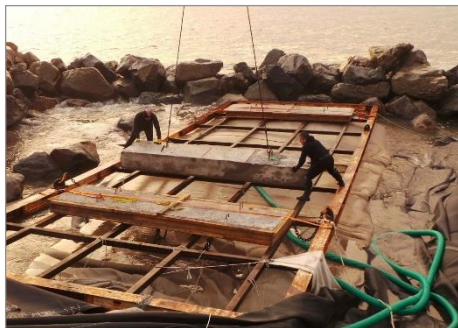
Figure 2: left: Initial filling of a tube; right: tube filling with diver support
