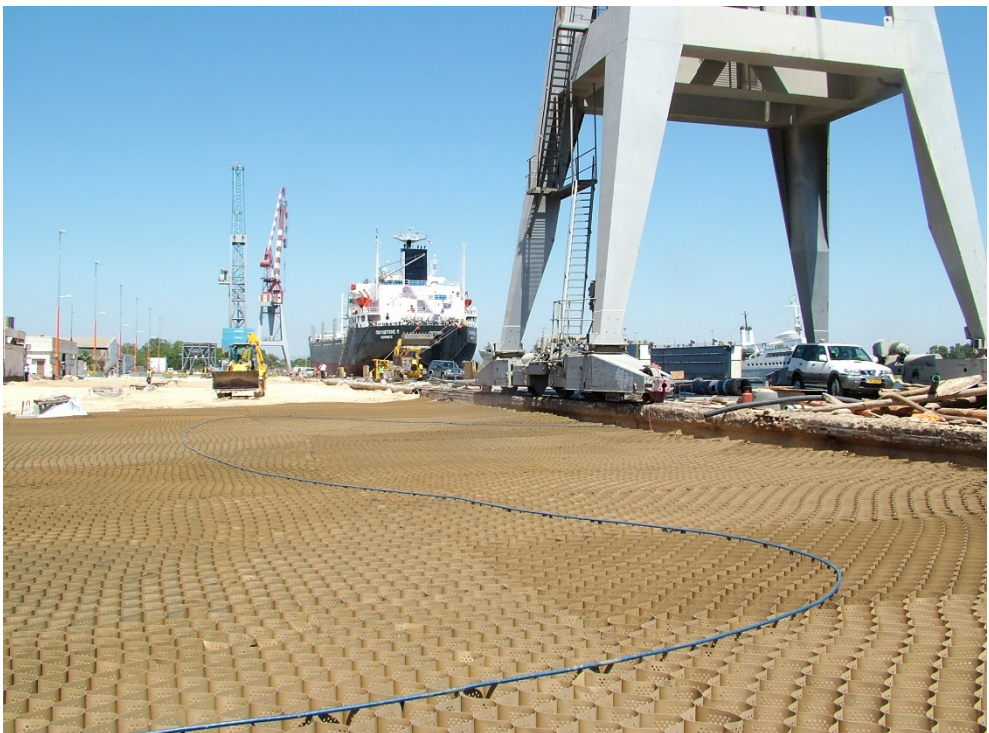
Figure 2: Heavy Loading Platform, Israel
