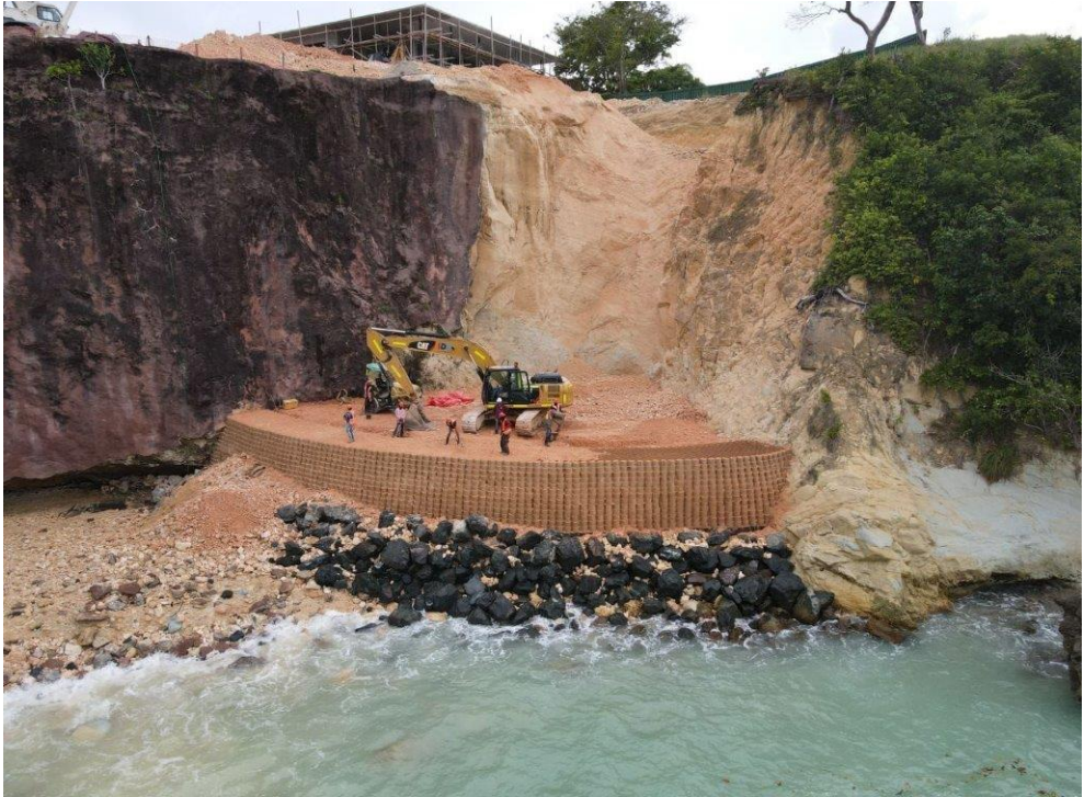
Figure 1: Retaining Wall, Dominican Republic
