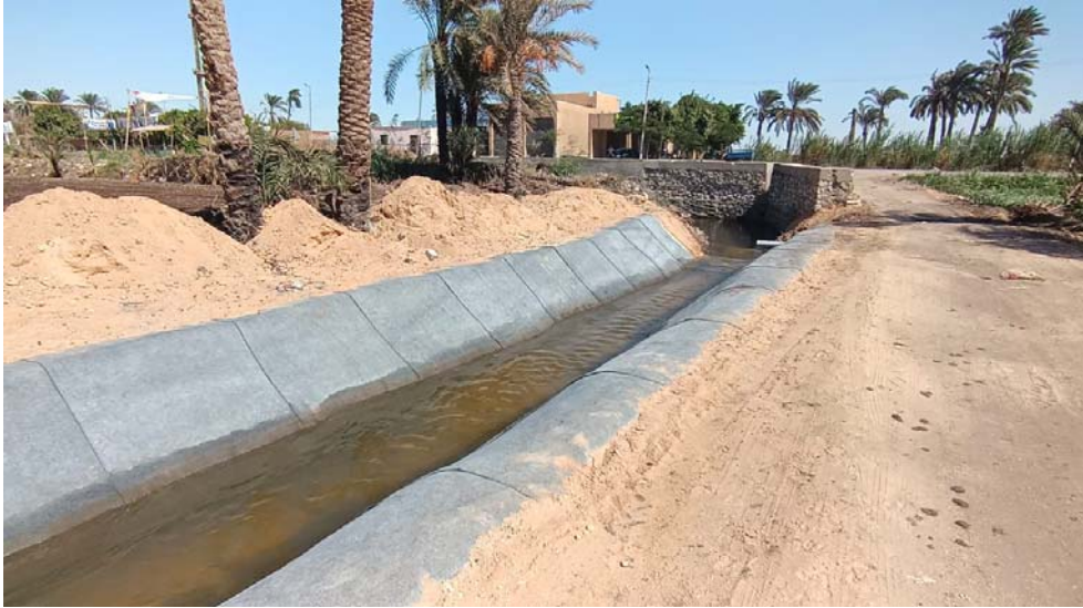
Fig. 1. Atfih, Egypt Type II GCCM canal lining trial at completion
