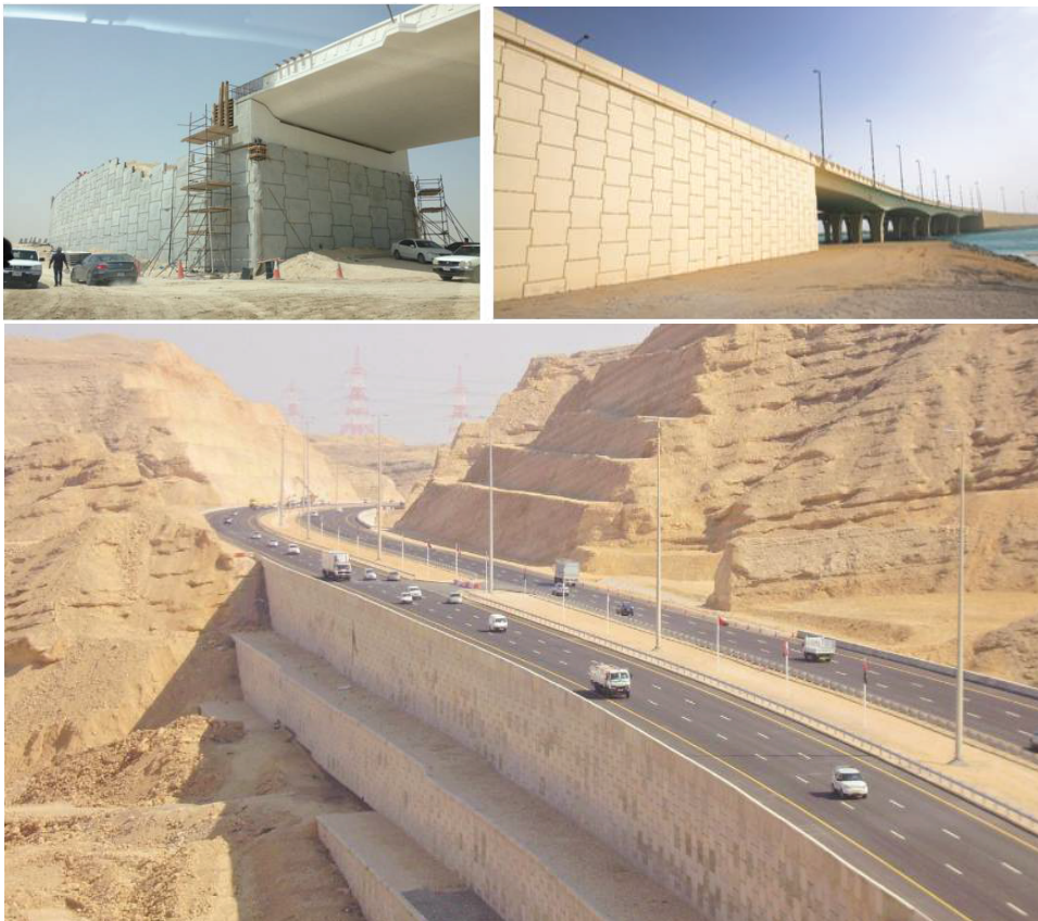
Fig. 2. Examples of polymeric strip reinforced soil walls and abutments in Middle East [7].
