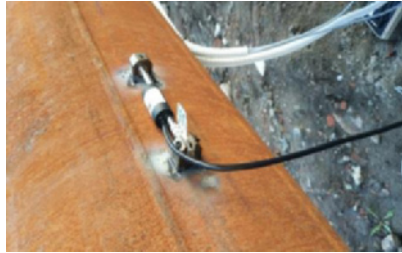
Fig. 2 View of the pit with struts and a mounted sensor.
