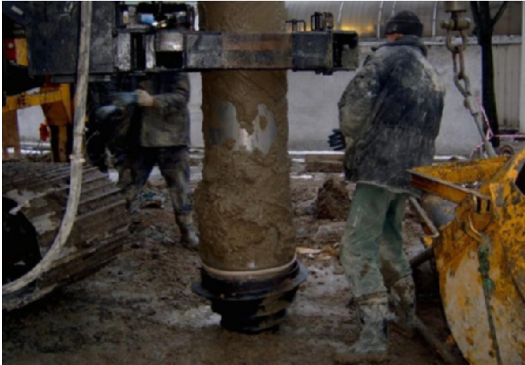
Fig. 2. The 350 mm diameter Fundex pile installation process.
