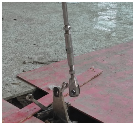
Figure. 7 Removal process of the vertical cable
