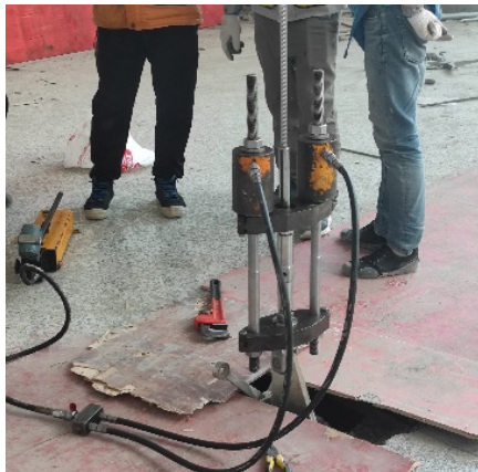
Figure. 7 Removal process of the vertical cable
