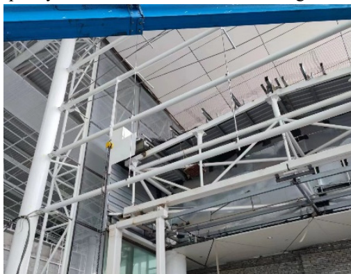
Figure .8 Removal process of self-balancing point support with cable structure
