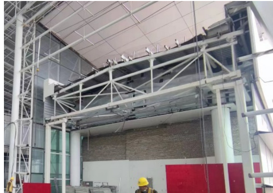
Figure .8 Removal process of self-balancing point support with cable structure
