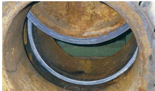
Fig. 10. Reconditioning of wedge gate.
