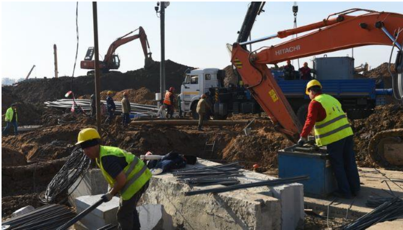
Fig. 3. The construction of wastewater treatment plants [3].
