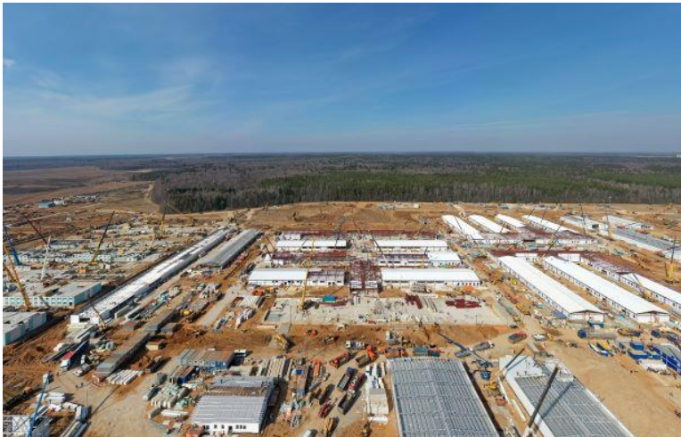
Fig. 2. Construction of the Moscow clinical center for infectious diseases [3].
