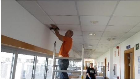
Fig. 6. On site application
