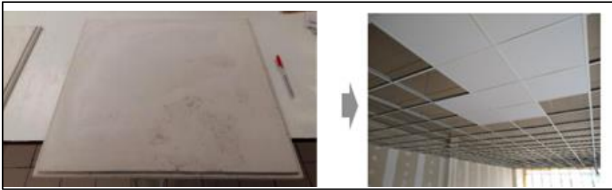
Fig. 3. Gypsum ceiling tile test piece (left), Gypsum ceiling tile installed in a ceiling (right).
