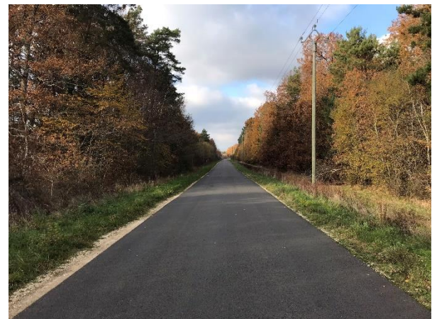
Fig. 6. Photo of adapted road by sealing its sides on December 9, 2022.
