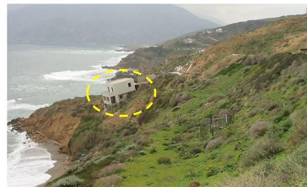
Fig. 3. Bassales landslide in Skiros island, North Aegean Sea, Greece. A landslide activated by heavy, prolonged rainfall, leading to large deformation causing the characteristic translation and rotation of the house in the ellipse.
