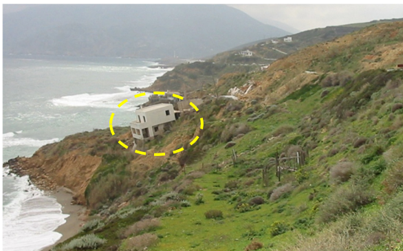
Fig. 1. Bassales landslide in Skiros island, North Aegean Sea, Greece. A landslide activated by heavy, prolonged rainfall, leading to large deformation causing the characteristic translation and rotation of the house in the ellipse.
