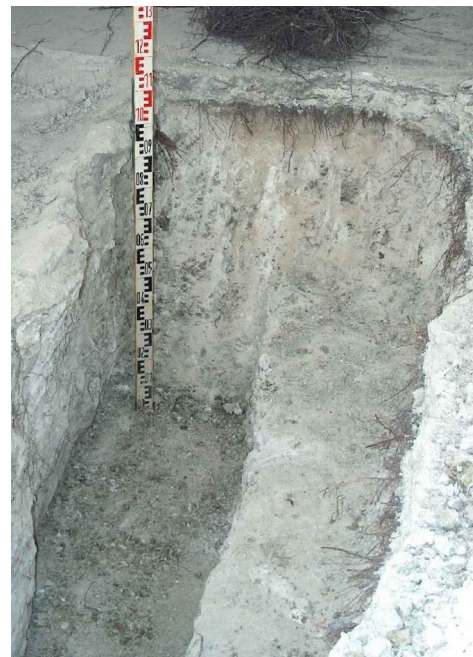
Fig. 6. Soil profile and roots system below the basement floor in trial pit T3.
