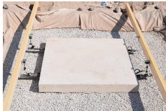
Fig. 7. View of the settlement monitoring arrangement.
