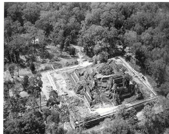
Fig.20 Failure of north-eastern side in 1943 [6]
