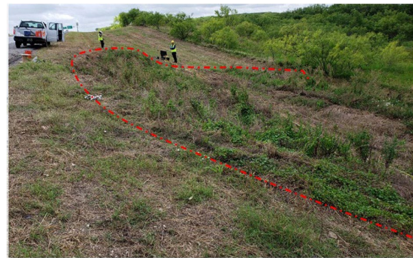
Fig. 1. Site condition after failure in 2019.
