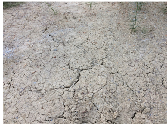
Fig. 1. Visible desiccation cracking at outcrop of very highly expansive Nicosia marl.
